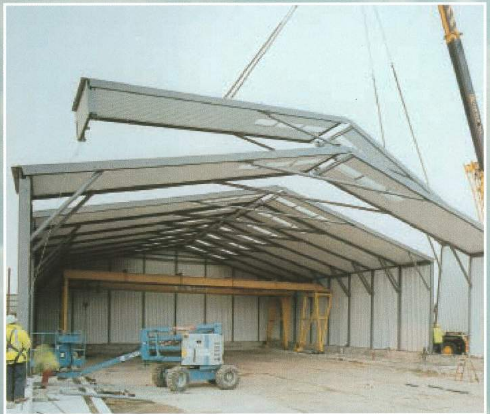
Pictures courtesy of Hy Ten Group Ltd. Quickway Q20 building x 38.2m erected in 12 days.
